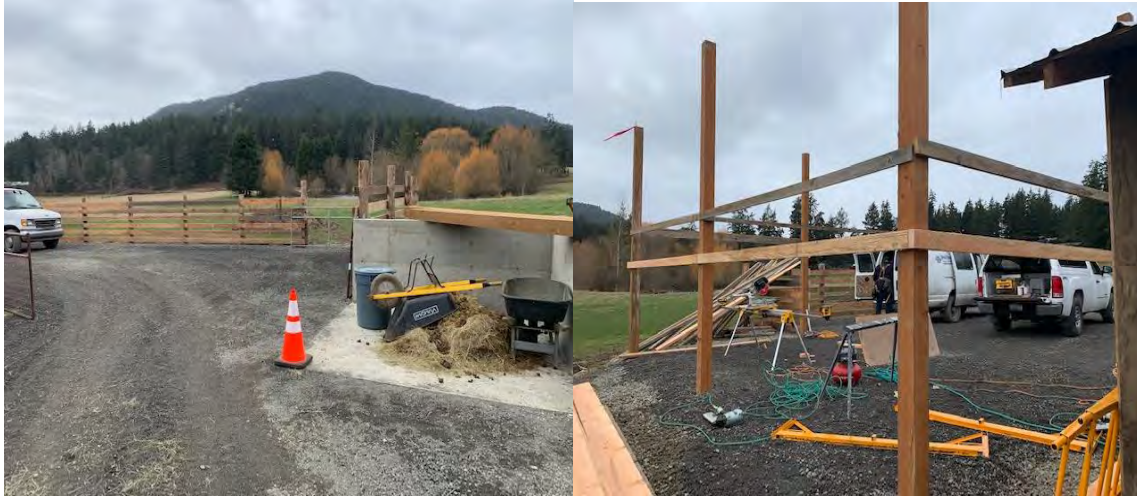
Photo 9. Coffelt compost shed foundation, new fencing and loafing shed frame
