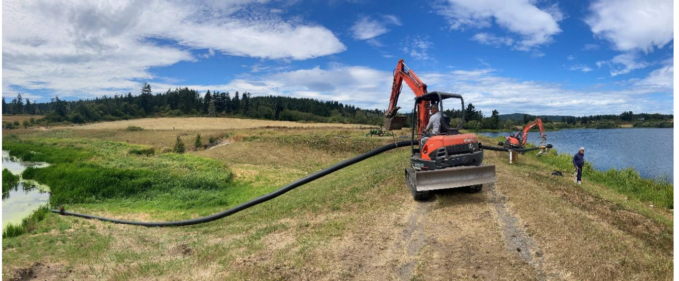
Photo 9. Eco Earthworks and Mainstay Marine midway into siphon installation at Zylstra
