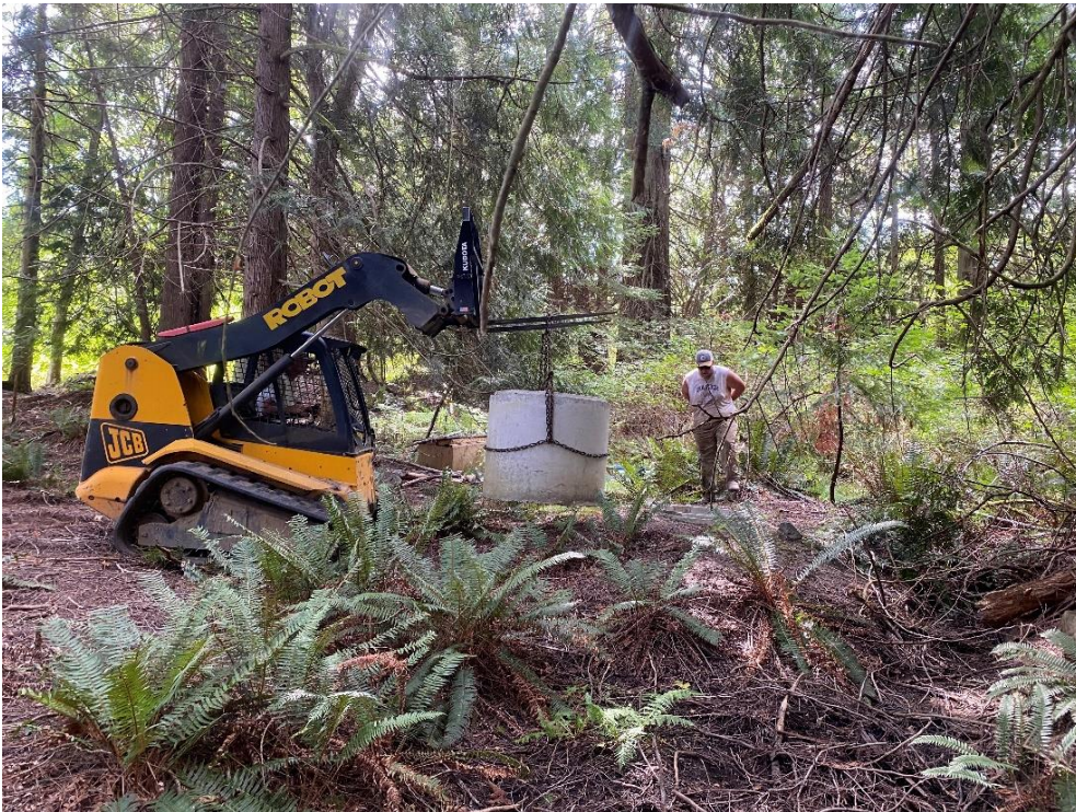
Photo 3. Decommissioning the dug well at the Lester cabin, Cady Preserve
