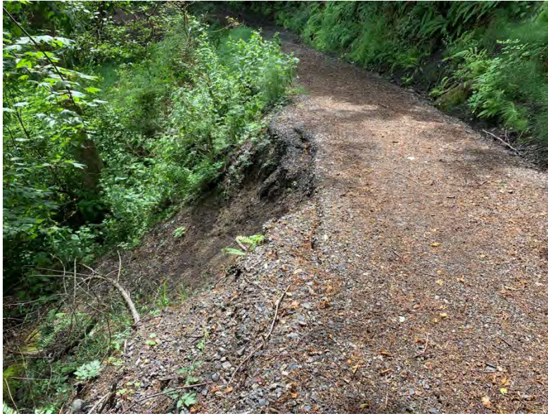
Photo 3. Slope failure requiring attention along the beach access road at the North Shore-Glenwood property.
