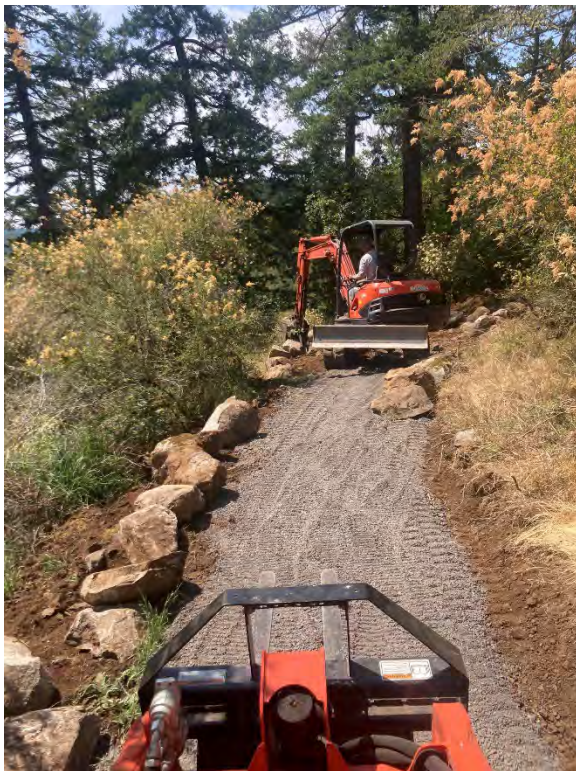
Photo 4. View from Kuby (our mini track loader) of EcoEarthworks building rock retaining wall at Beaverton Marsh Viewpoint
