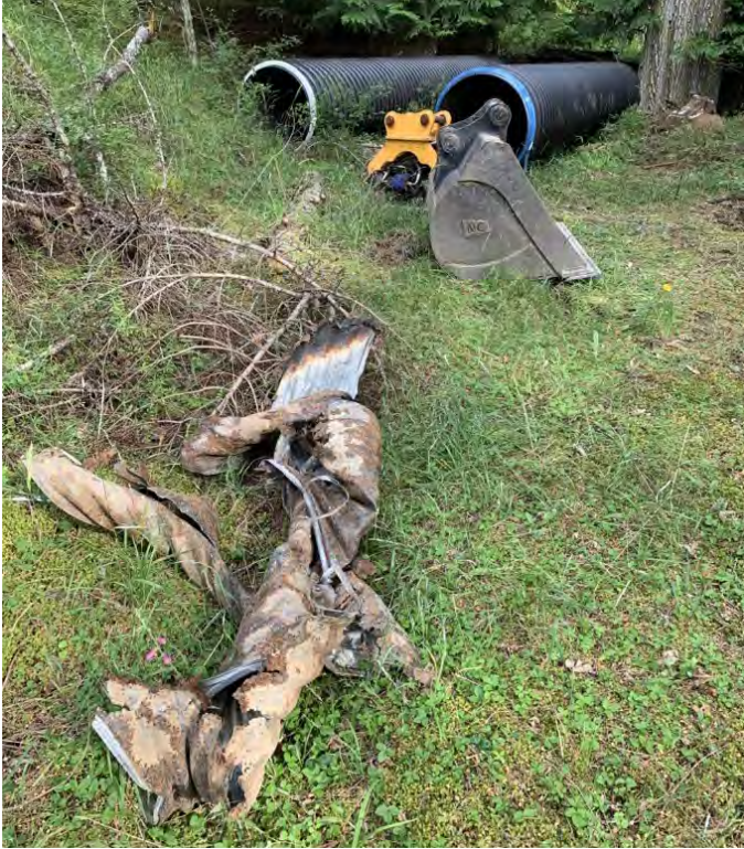
Photo 7. Turtleback culverts. Before (old culvert in foreground).
