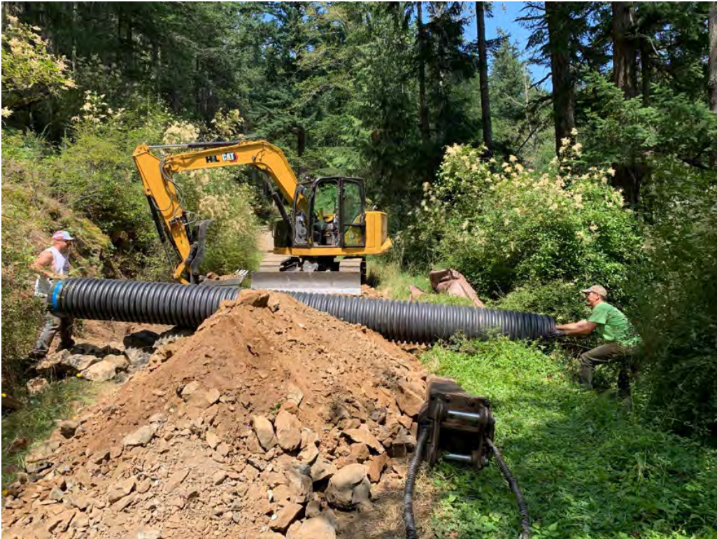
Photo 8. Turtleback culverts. One of 20.
