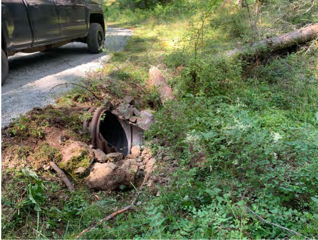
Photo 9. Turtleback culverts. New culvert buttoned up.
