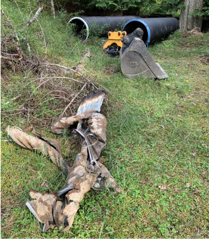
Photo 7. Turtleback culverts. Before (old culvert in foreground).
