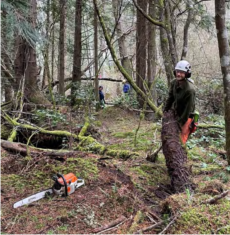
Photo 13. Trail work at Spencer Spit Preserve, with Andrew, Shauna and Jacob.
