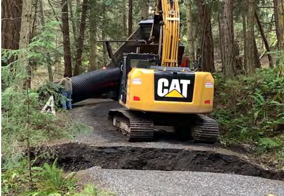
Photo 7. Culvert replacement at Turtleback Mountain Preserve.
