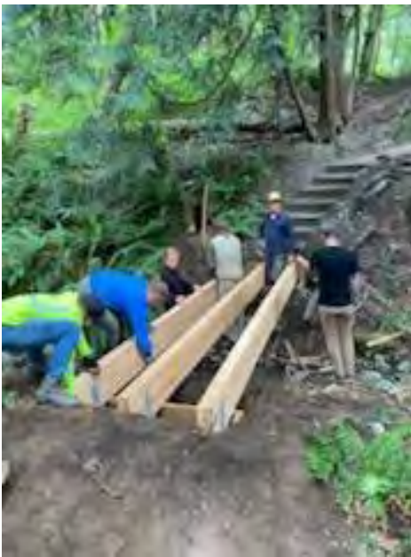
Photo 4. Turtleback bridge replacement under way.
