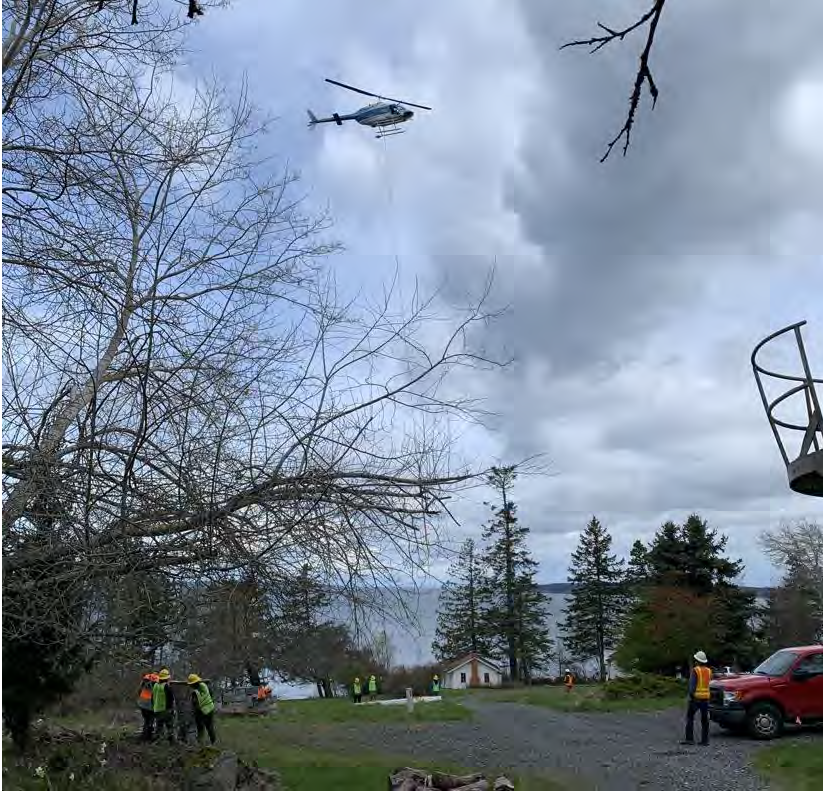
Photo 12. DNR helicopter lift of Point Doughty restroom building materials.
