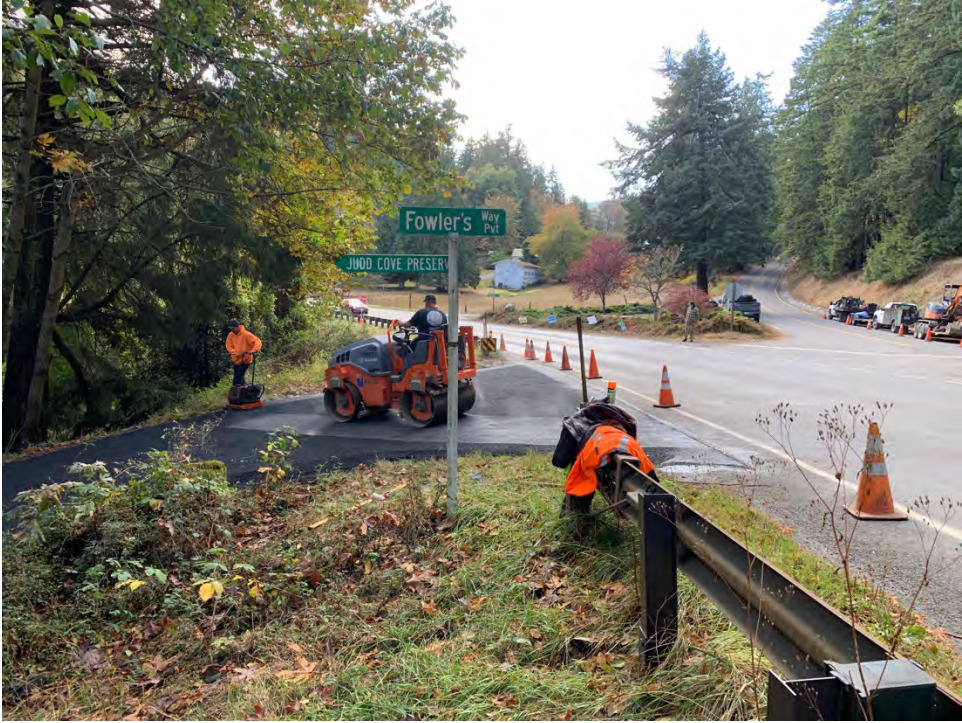
Photo 3: Contractor wraps up paving at the entrance to Judd Cove Preserve.
