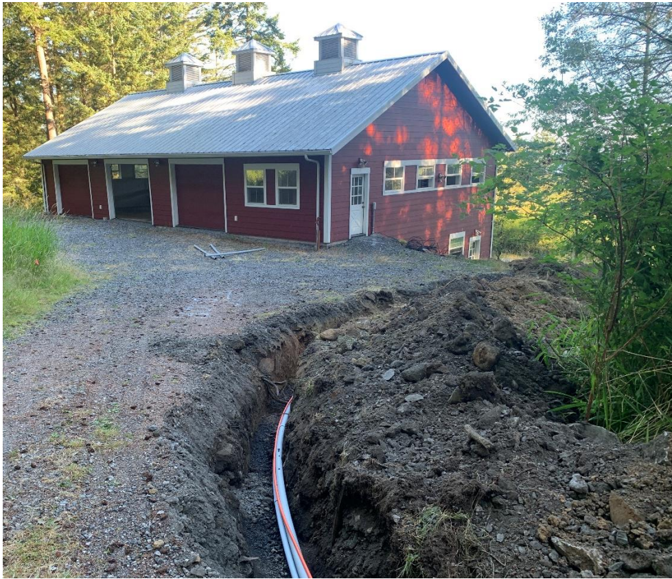
Photo 7. New electrical and water lines were installed to the North Shore garage.
