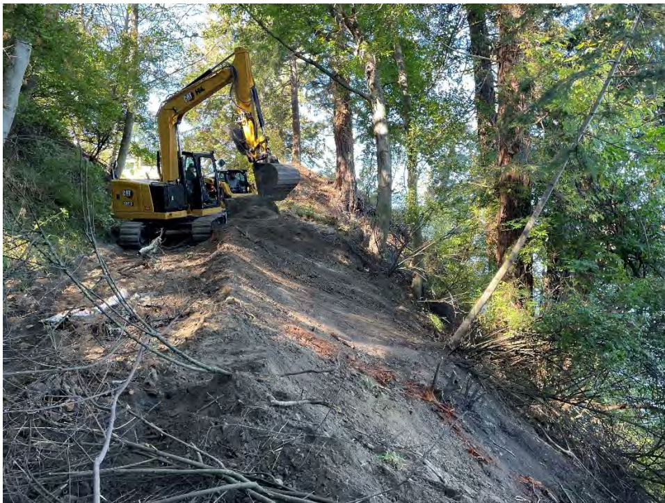
Photo 12. Preliminary grading of the old road to remove slide material, North Shore Preserve.
