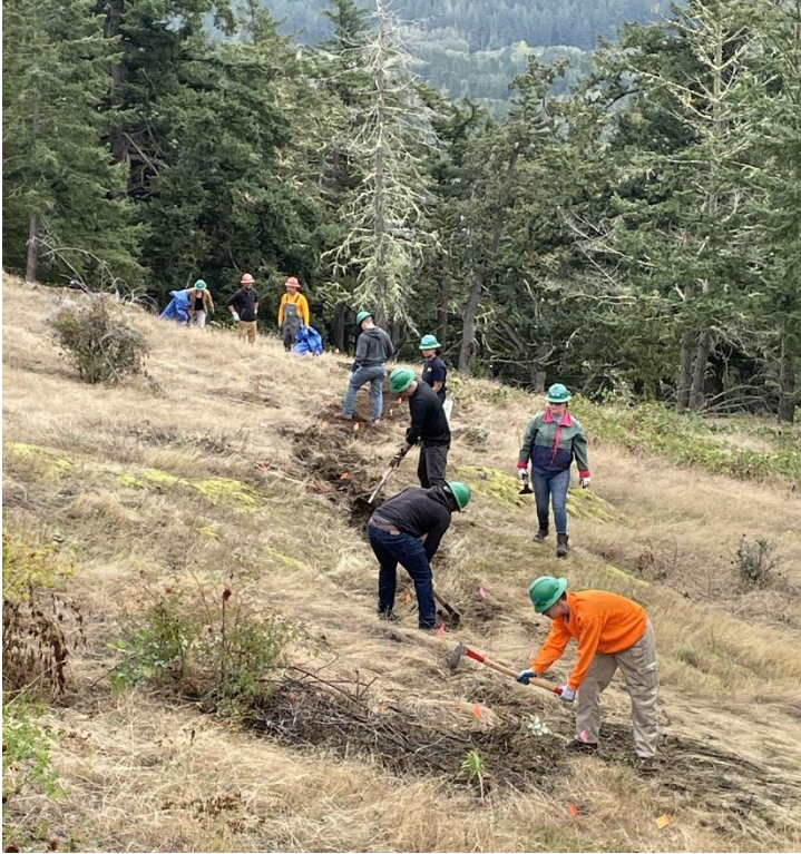
Photo 15. A crew from WTA realigns the upper Morning Ridge Trail, Turtleback Mountain Preserve.
