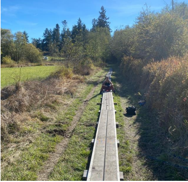
Photo 7: Shauna “testing” out the newly installed bog bridge, Zylstra Lake Preserve
