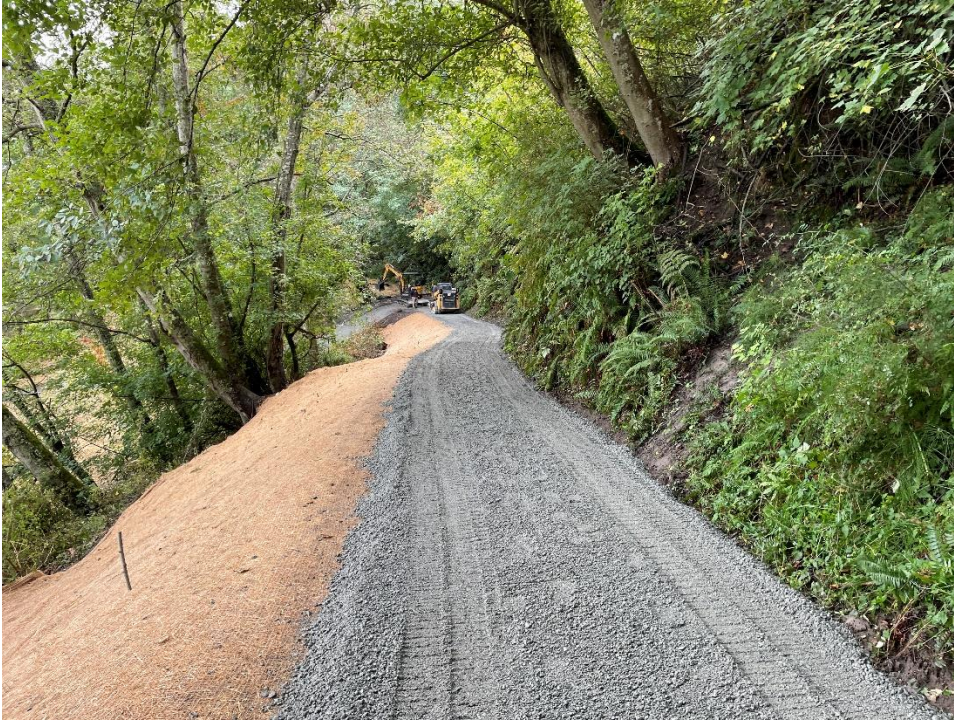
Photo 13. Finishing up the road-to-trail conversion and establishing erosion control, North Shore Preserve.
