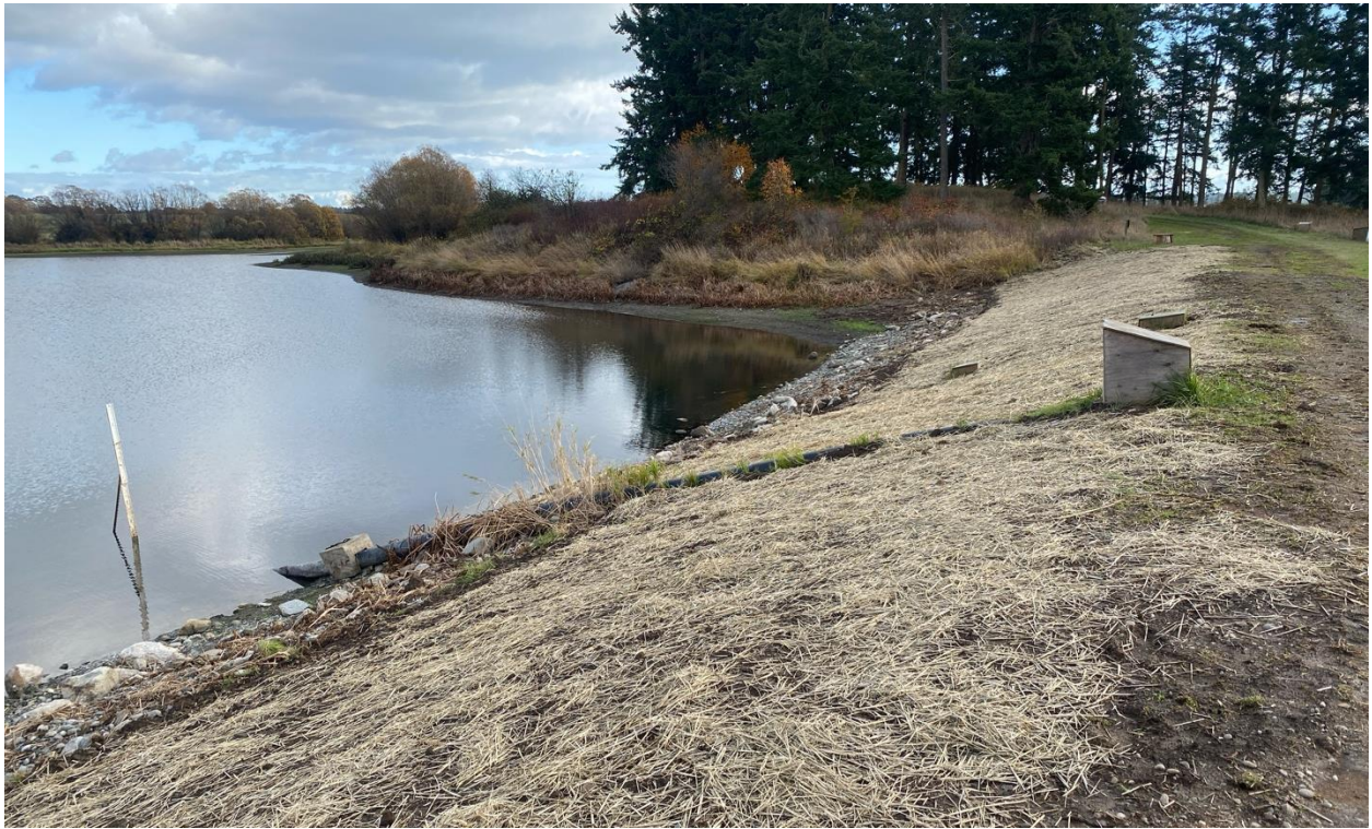
Photo 6. Contractors filled in animal burrows and smoothed the face of the upper dam, Zylstra Lake Preserve.
