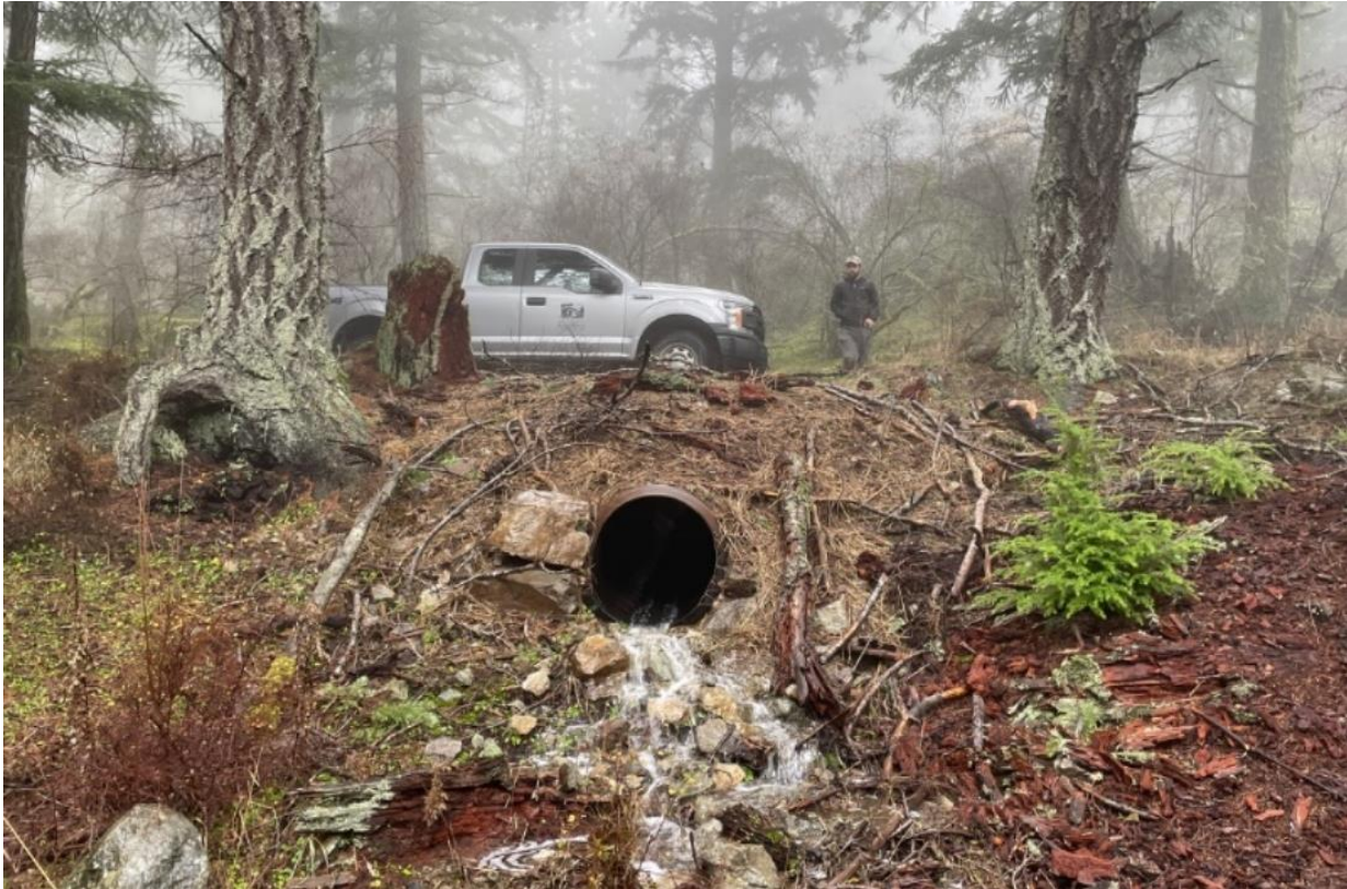
Photo 17. Staff inspect one of 20 new culverts following heavy rains. Several culverts returned flow to seasonal streams that'd been dry since the road was installed many decades ago, Turtleback Mountain Preserve, Orcas.
