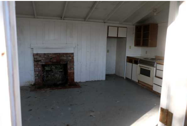
Living room, kitchen and brick fireplace; view to the southwest.
