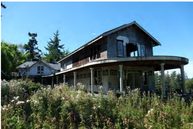
c.2010 wing with original house in background; view to the southwest.
