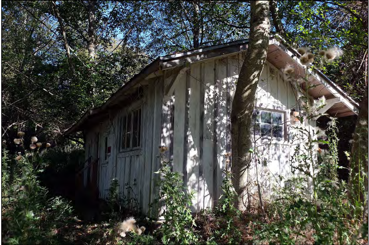
Figure 66: East cottage at top of bluff; view to the east.
