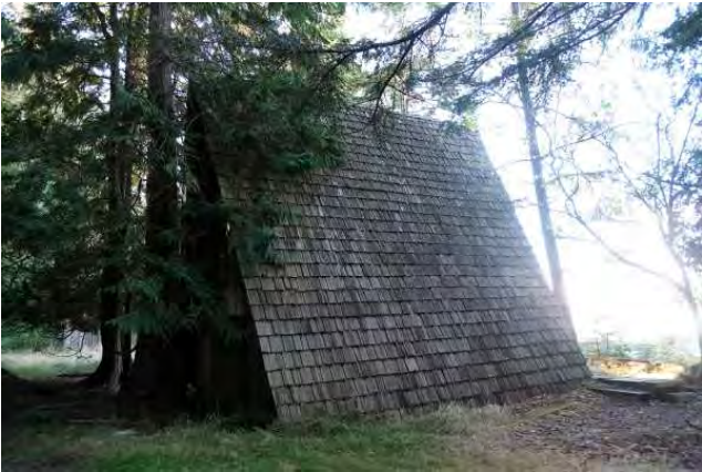
Southeast corner of A-frame; view to the northwest.
