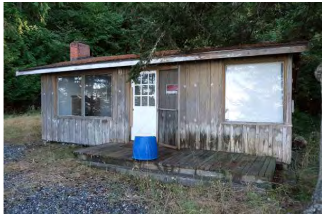
North side of cottage; view to the south.
