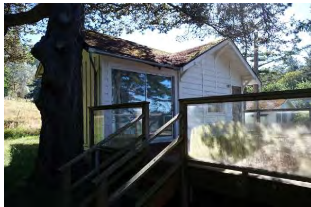
North side of cottage, showing deck and sliding glass door; view to the southwest.
