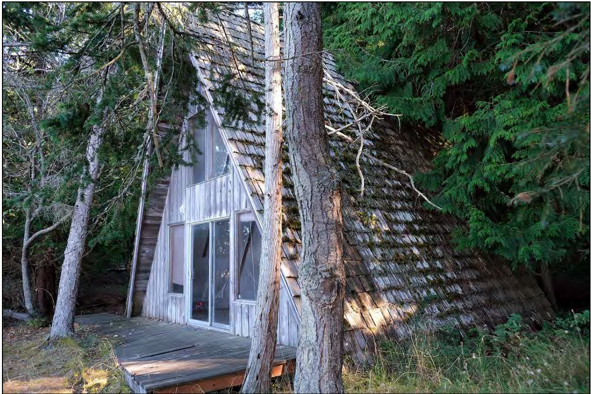
Figure 67: A-frame on beach; view to the southeast.
