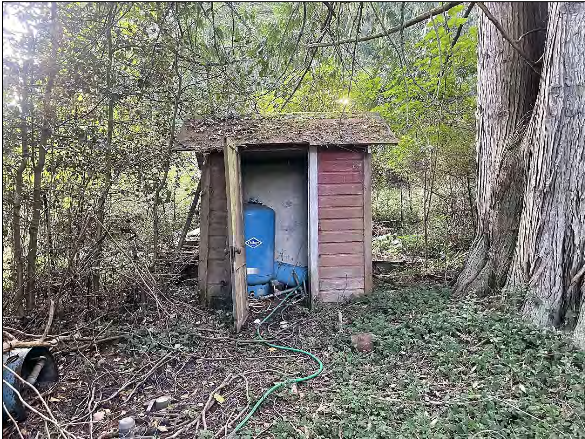
Figure 70. Pump house with concrete spring box behind it; view to the east.
