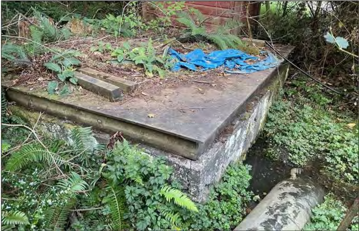
Figure 26: Spring box and east wall of adjacent pumphouse, view west-southwest.
