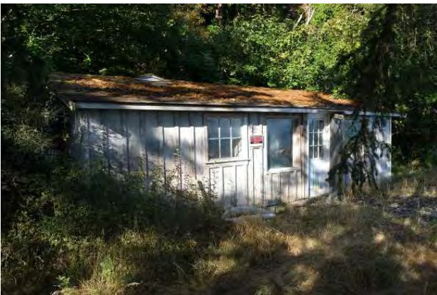
North side of cottage; view to the southwest
