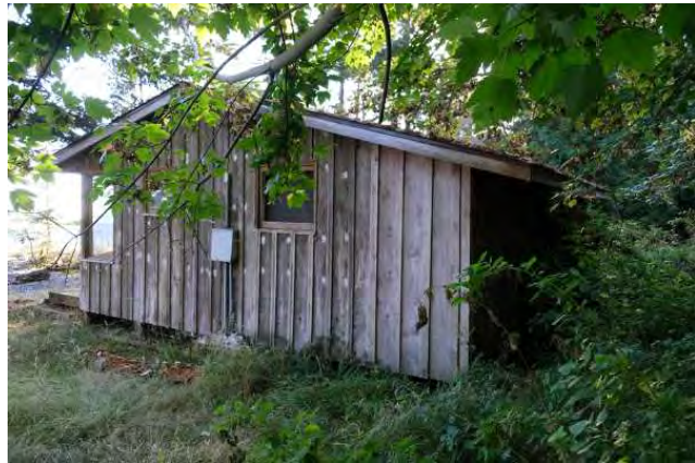
West wall of cottage; view to the northeast
