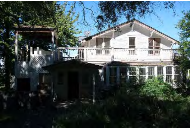
South wall of house, showing first floor extension, balcony and two-story gazebo; view to the north.
