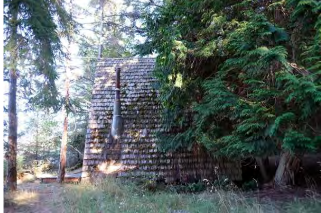
West side of A-frame; view to the east
