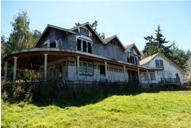
Main house with c.2010 addition in foreground; view to the southwest.
