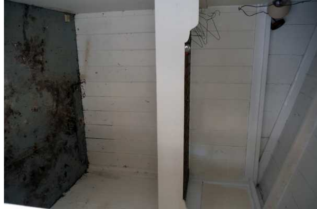
Built-in bunk bed in cottage; view to the east.
