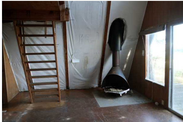
Interior of A-frame, showing ladder and fireplace; view to the west.
