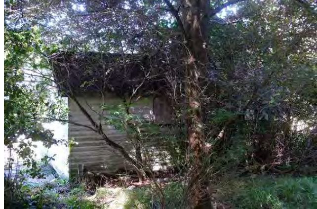
South side of cottage; view to the northeast.
