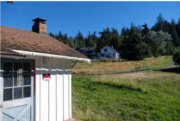
View southeast to main house from cottage.
