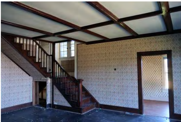
North room and stairway, view to the southwest.
