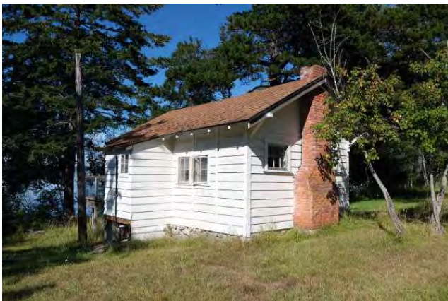
Southwest corner of cottage; view to the northeast.
