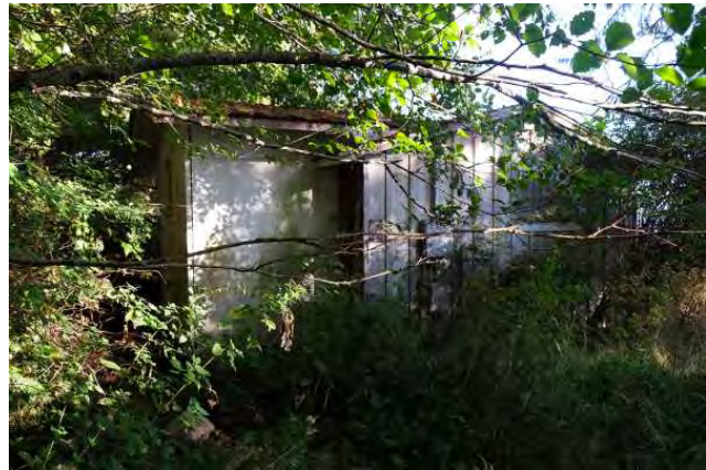
Southeast corner of building; view to the northwest.
