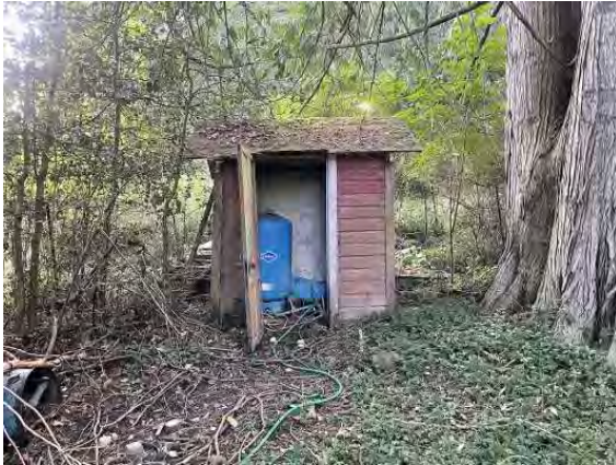
Pump House, view to the east
