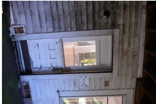
East door, viewed from east porch; view to the west.
