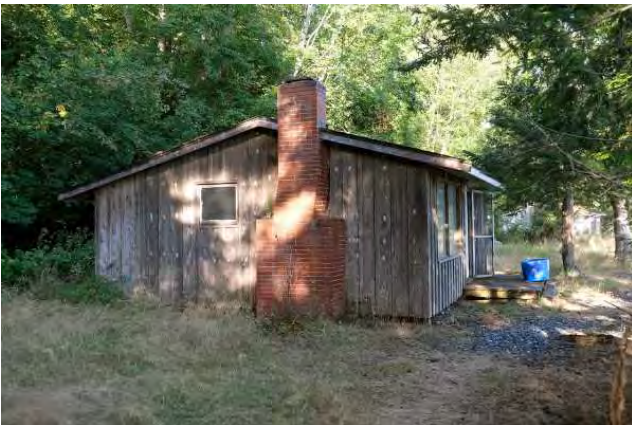
East wall of cottage, showing brick chimney; view to the southwest.
