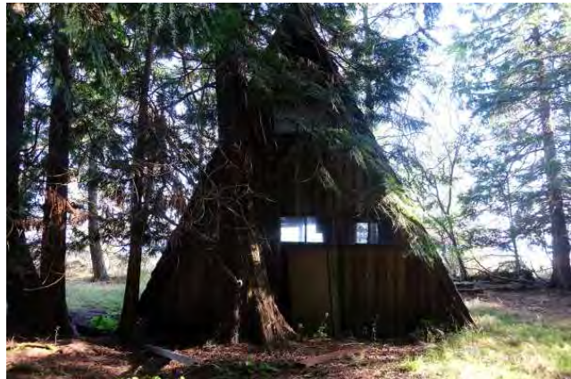
Back (south) side of A-frame; view to the north.
