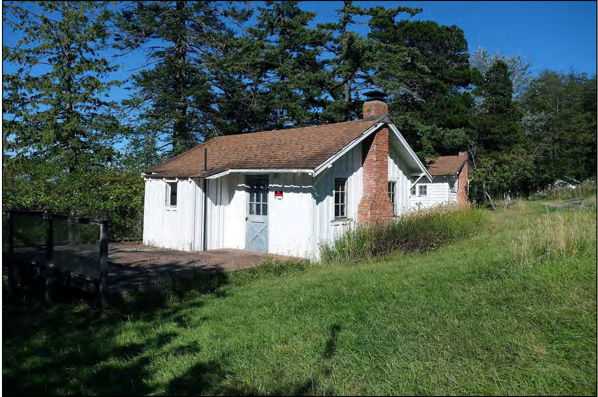
Figure 64: West cottage at top of bluff; view to the northeast.
