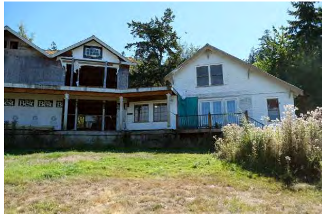
Main house: junction of original house and c.2010 addition; view to the south.
