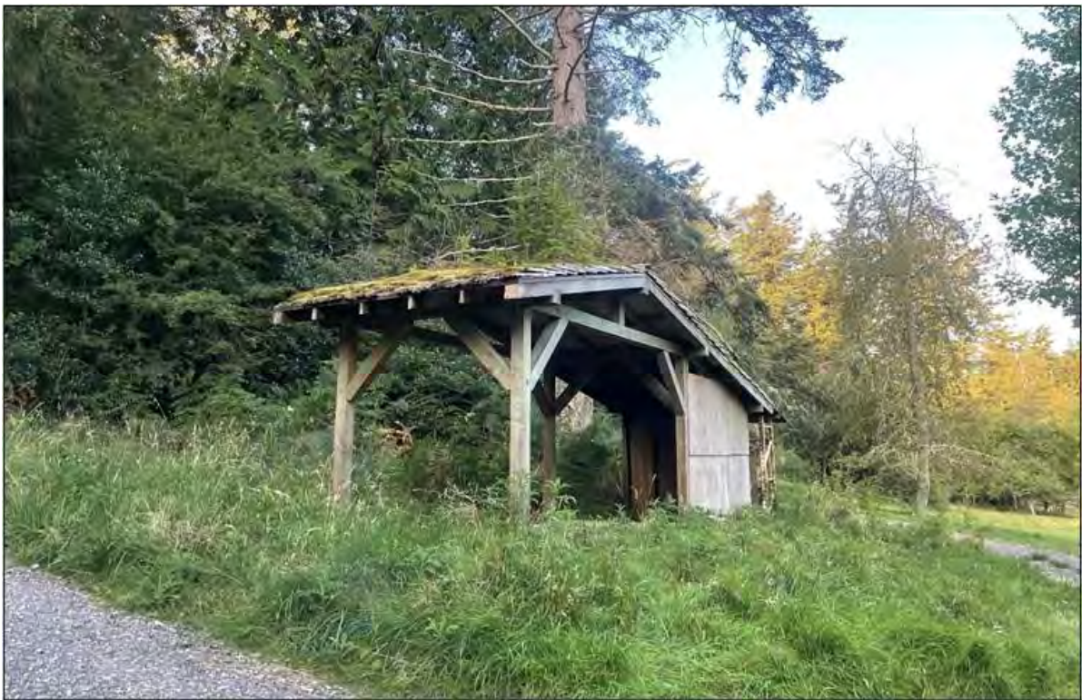
Figure 25: View southwest, woodshed.
