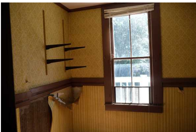
Two-over-two double-hung sash window in south gable; view to the south.
