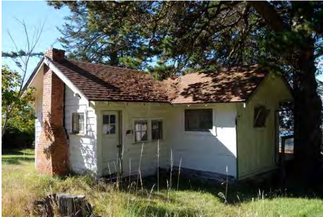
Cottage, view to the northwest.
