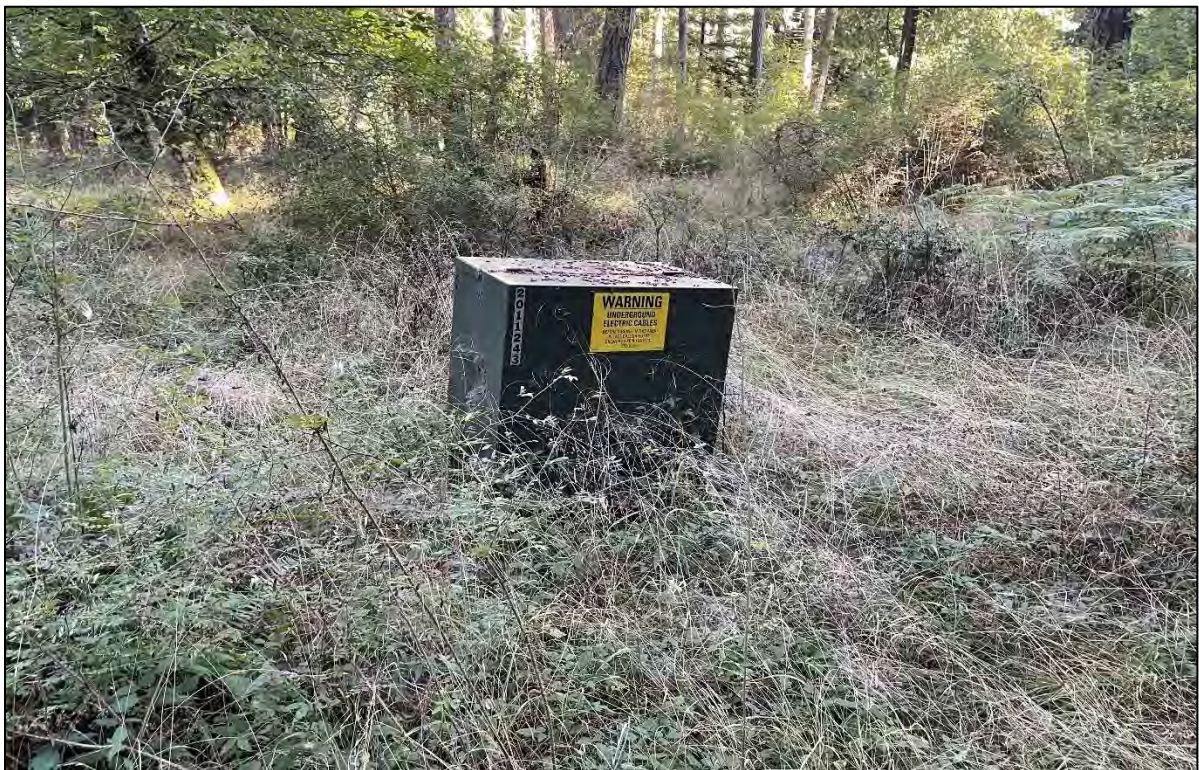
Figure 33: View northeast, electrical box along utility corridor.
