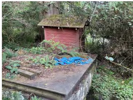
Pump house and spring box, view to the southwest.
