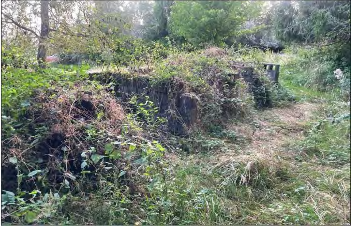
Figure 24: View northeast, northeast-most cinderblocks.
