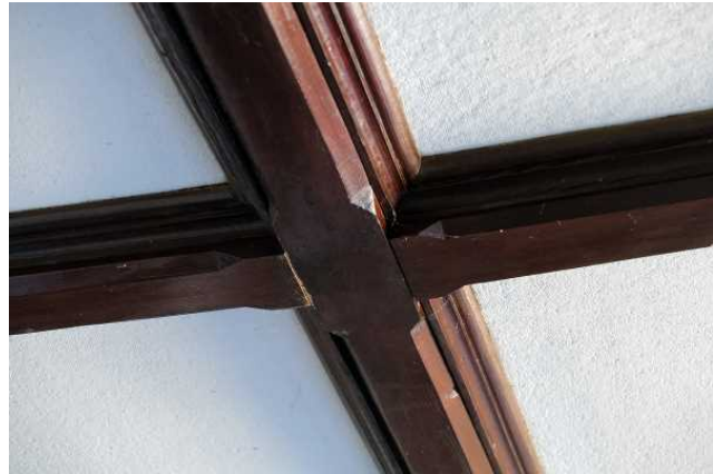
Ceiling beams in north room; view to the southwest.
