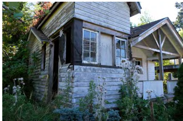
Two-story addition at northeast corner of cottage; view to the southwest.
