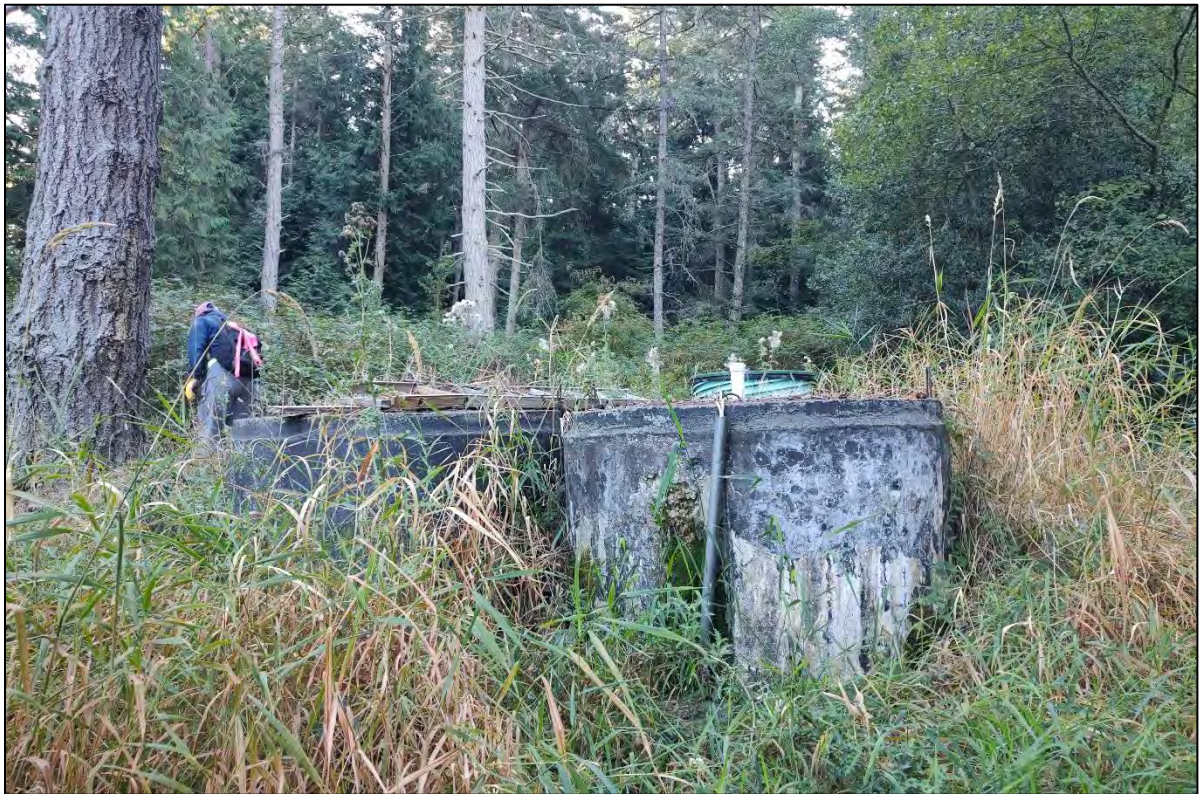
Figure 37: View southeast, overview of concrete tanks.
