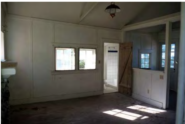
Cottage interior showing living room and kitchen (behind half wall); view to the northwest.
