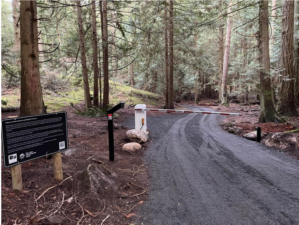
Photo 4. The Land Bank's first automated entry gate at the North Shore Preserve will allow dawn to dusk access by future preserve users, while enabling the neighbor to reach their property (via an easement) using remote openers.
