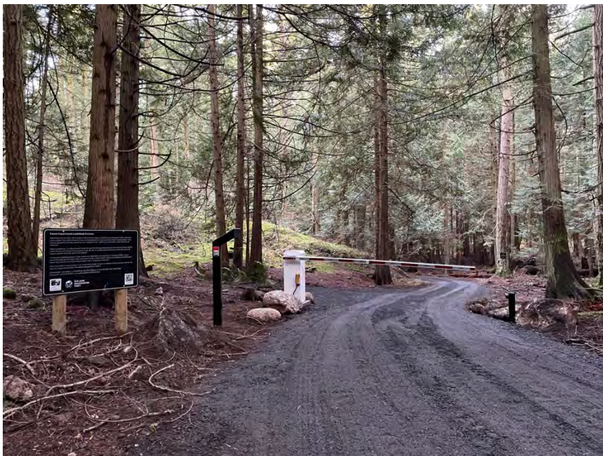
Photo 9. Automated gate at North Shore
