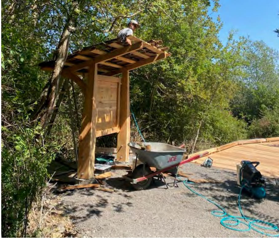
Photo 5. Jacob finishes the kiosk at the Linde-Beaverton trailhead.
