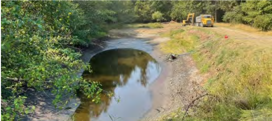
Photo 13. The pond was drawn-down in preparation for the wetland resotration project, at North Shore.
