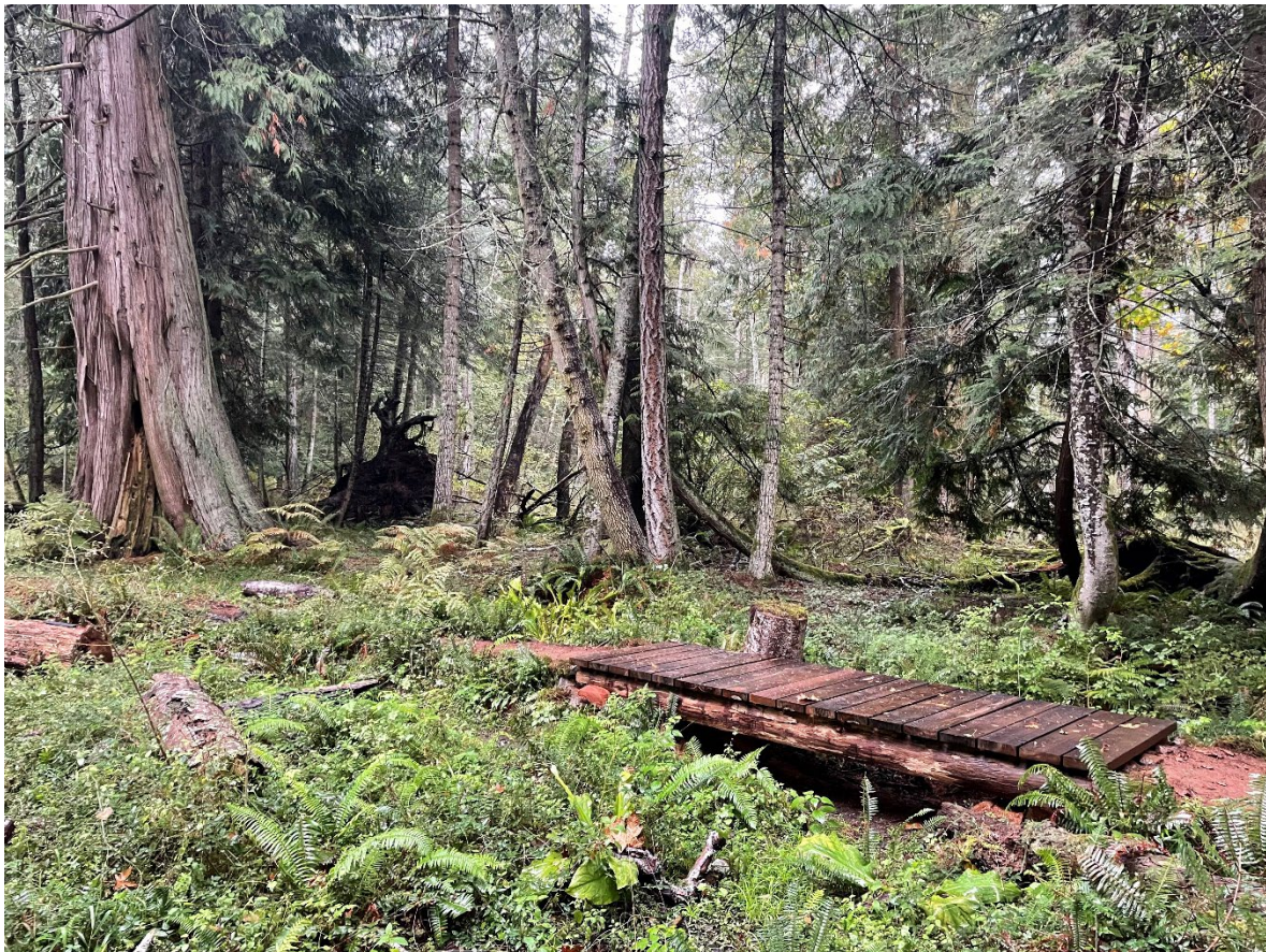
Photo 14. A stream-crossing is complete at Lopez Hill Preserve.
