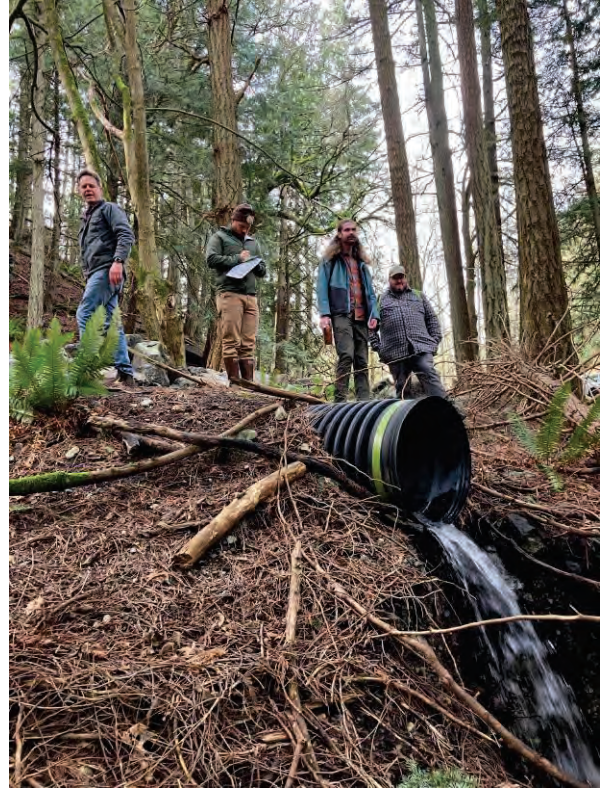
Photo 12. Staff led a field trip to review a grant proposal to restore the stream and wetland at Judd Cove Preserve. One component of the application is to remedy this perched culvert which erodes the hillside below and delivers high energy flow into wetlands.
