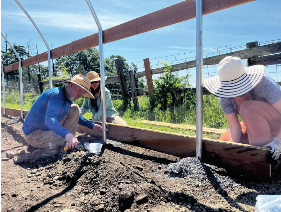
Photos 3. The greenhouse takes shape at the Salish Seeds Project nursery.
