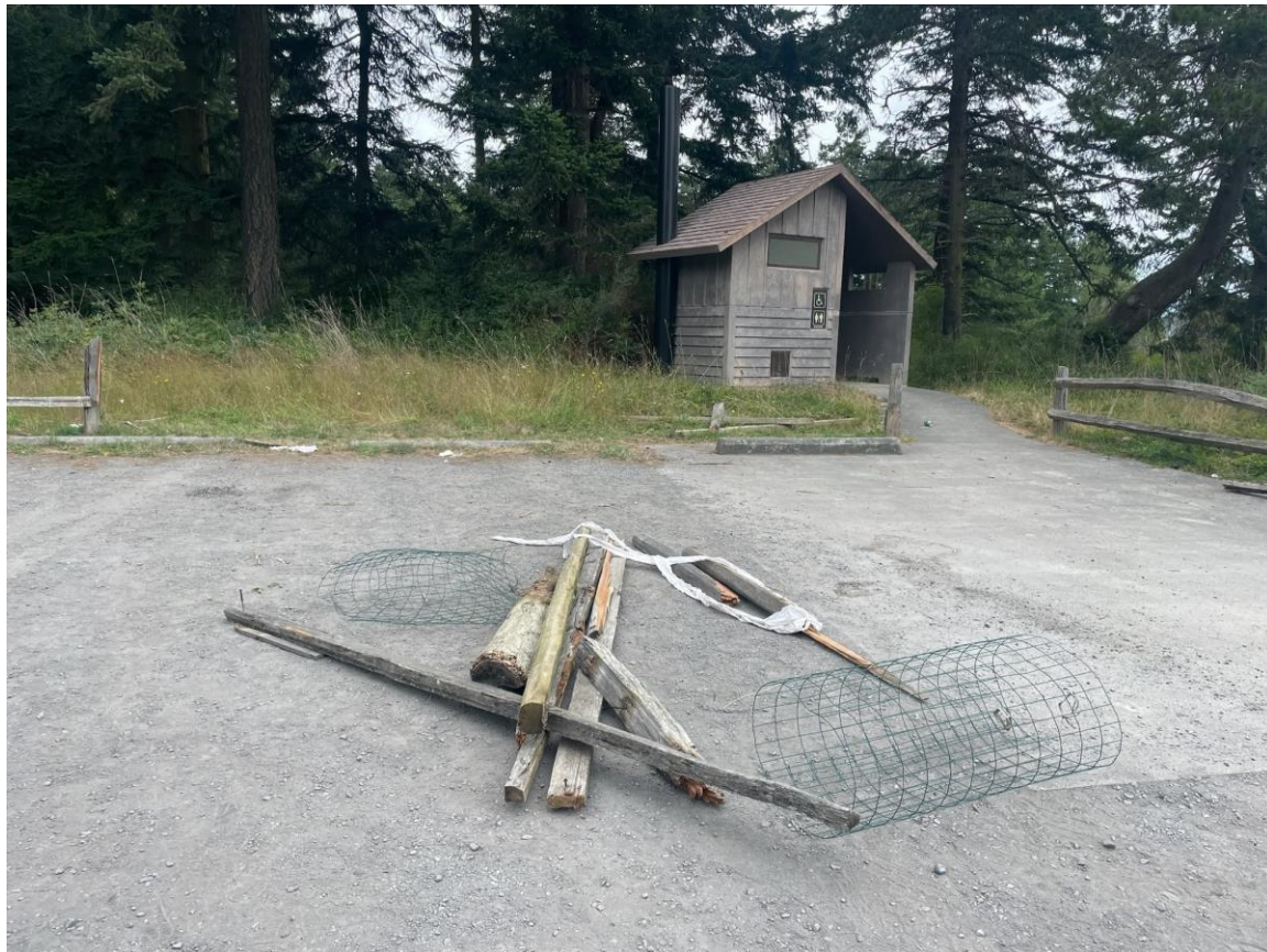
Photo 11. Damage to the Fisherman Bay Spit fence around the parking area.
