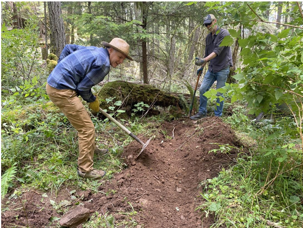
Photo 13. Peter and Scot prepare to lay a culvert under the trail at Turtleback Mountain Preserve.
