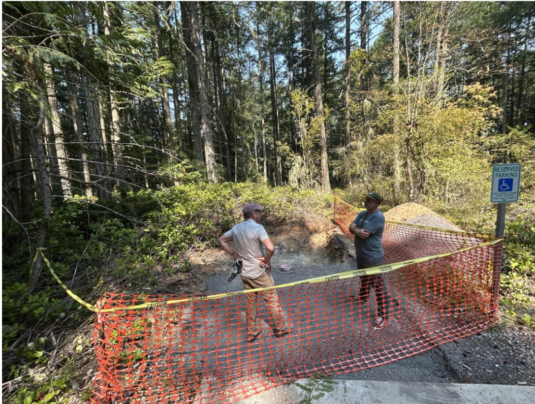
Photo 6. Doug and Pete contemplate the new restroom installation at Mount Grant Preserve.
